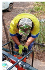
Leroy attaching pump to water fill point tank
